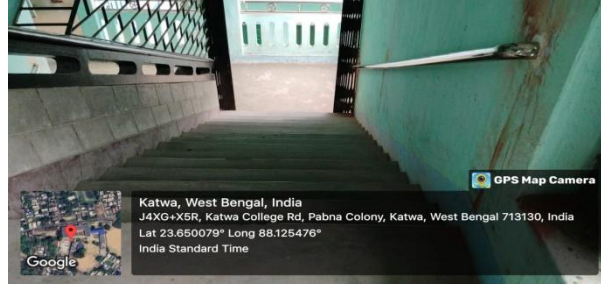
Installation of hand Railings in the staircases
